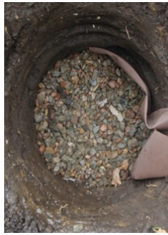
Add aggregate to drain sump hole (Optional) to reduce freeze/thaw heaving. Aggregate can also be added around drain sump sides when back-filling
