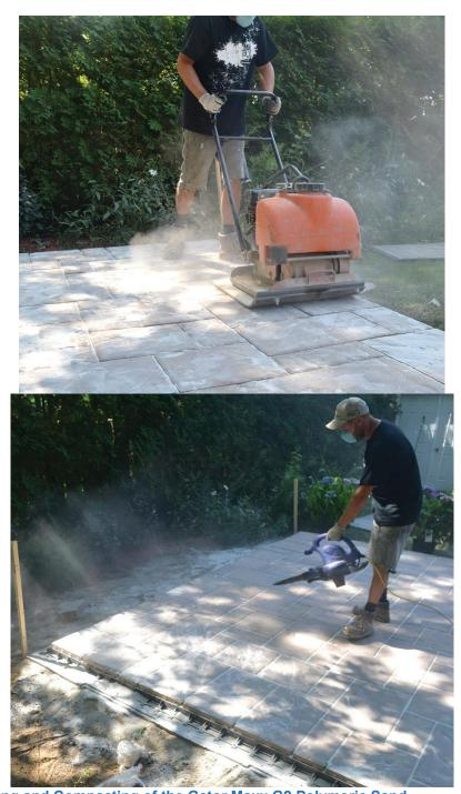
**STEP 6 • Sweeping and Compacting of the Gator Maxx G2 Polymeric Sand A •** When emptying the GATOR MAXX G2 polymeric sand bags, spread it onto the dry paved surface. This will avoid segregation and sweeping a mountain of sand. • When sweeping the polymeric sand, spread over a small area before moving onto the next, while making sure to fill in the joints.
