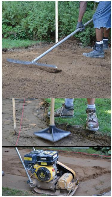
STEP 2 • Levelling and compacting of the subgrade
