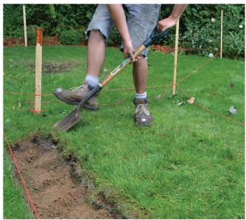
**STEP 1 • Excavation of the New Gator Base Area**
