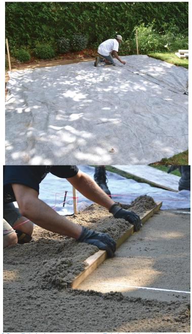
STEP 3 • Addition of Geo-Fabric (non-woven Gator Fabric 4,4) levelling and compacting bedding sand
